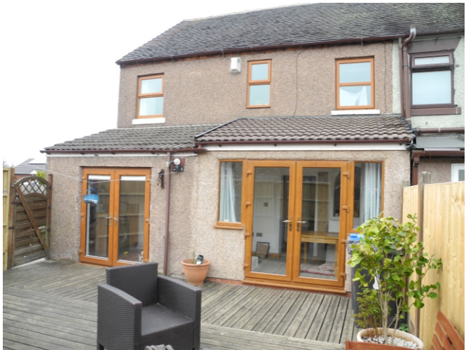
view of rear showing existing ground floor extensions
