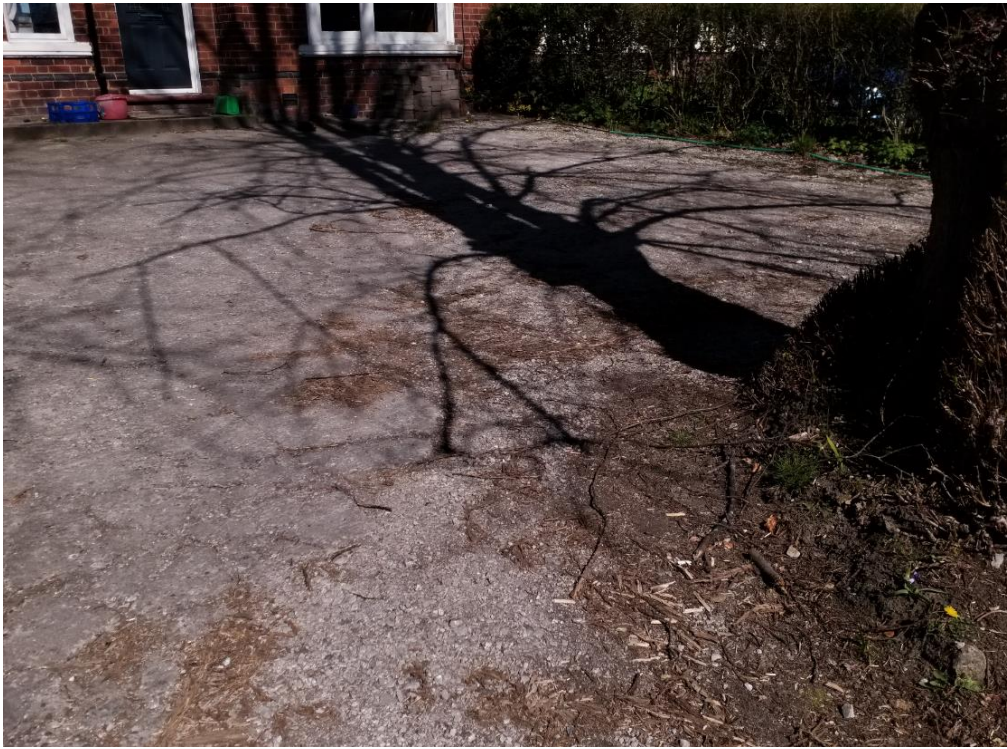
Fig 10: The concrete and hardcore driveway surface.
