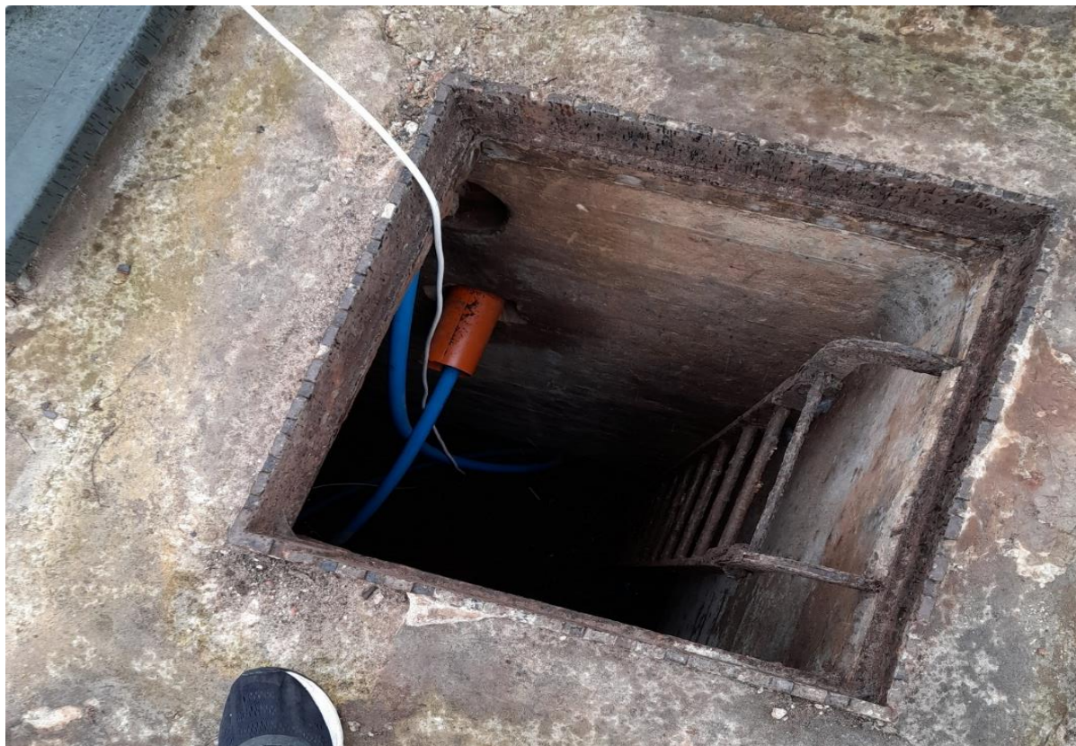
Plate 5: Image of the current entrance to the underground water tank.
