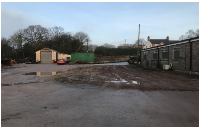
Existing Buildings on Site
