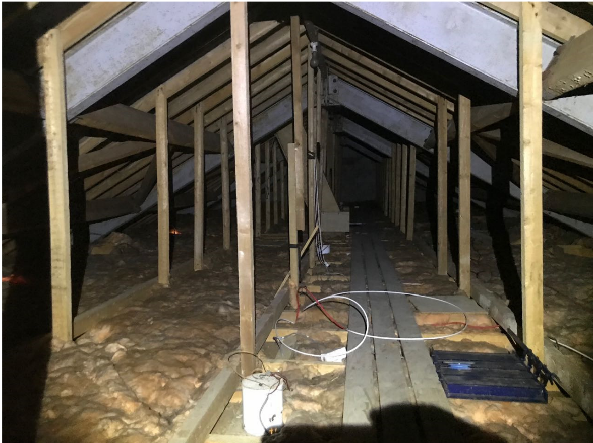
Roof void of Wedding Venue – central vertical support timbers to be removed to enable uncluttered environment for flying
