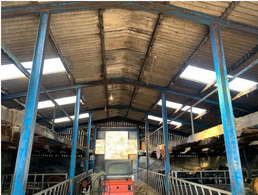
General internal view of larger portal frame with minor surface corrosion
