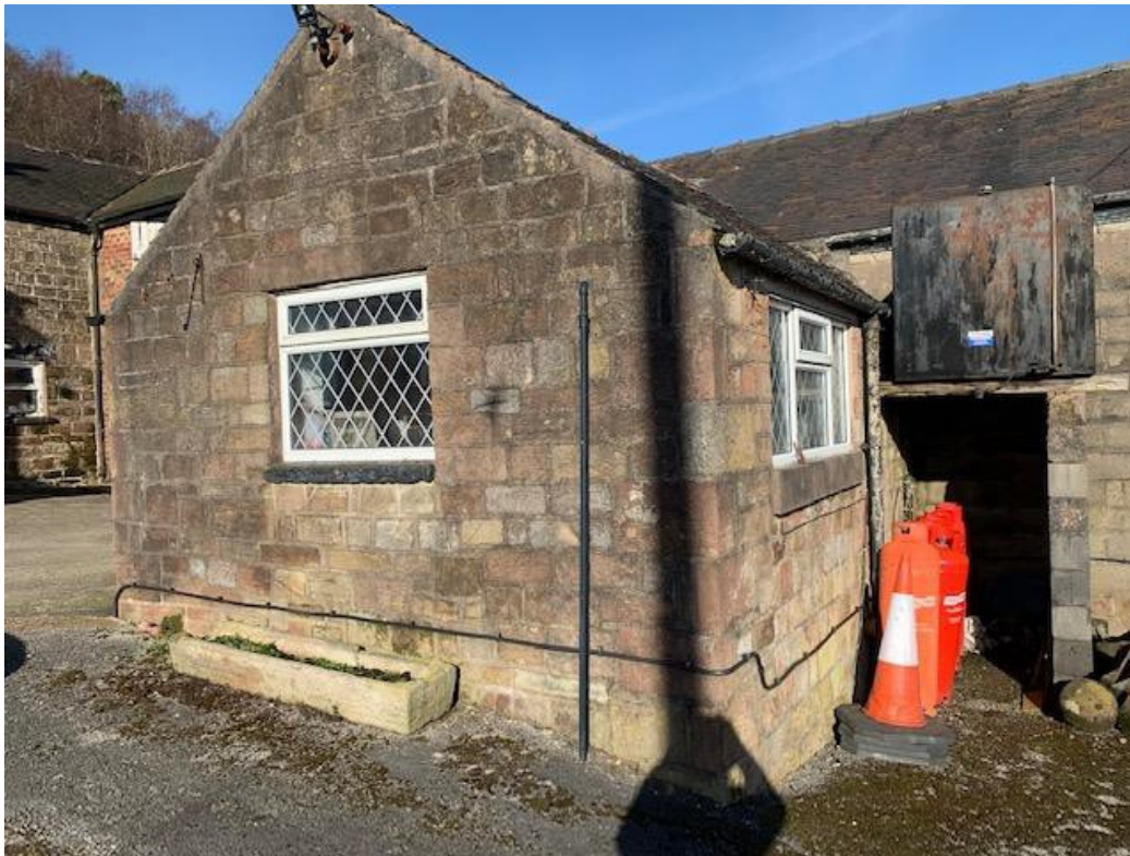
Small outrigger outbuilding in good structural condition.
