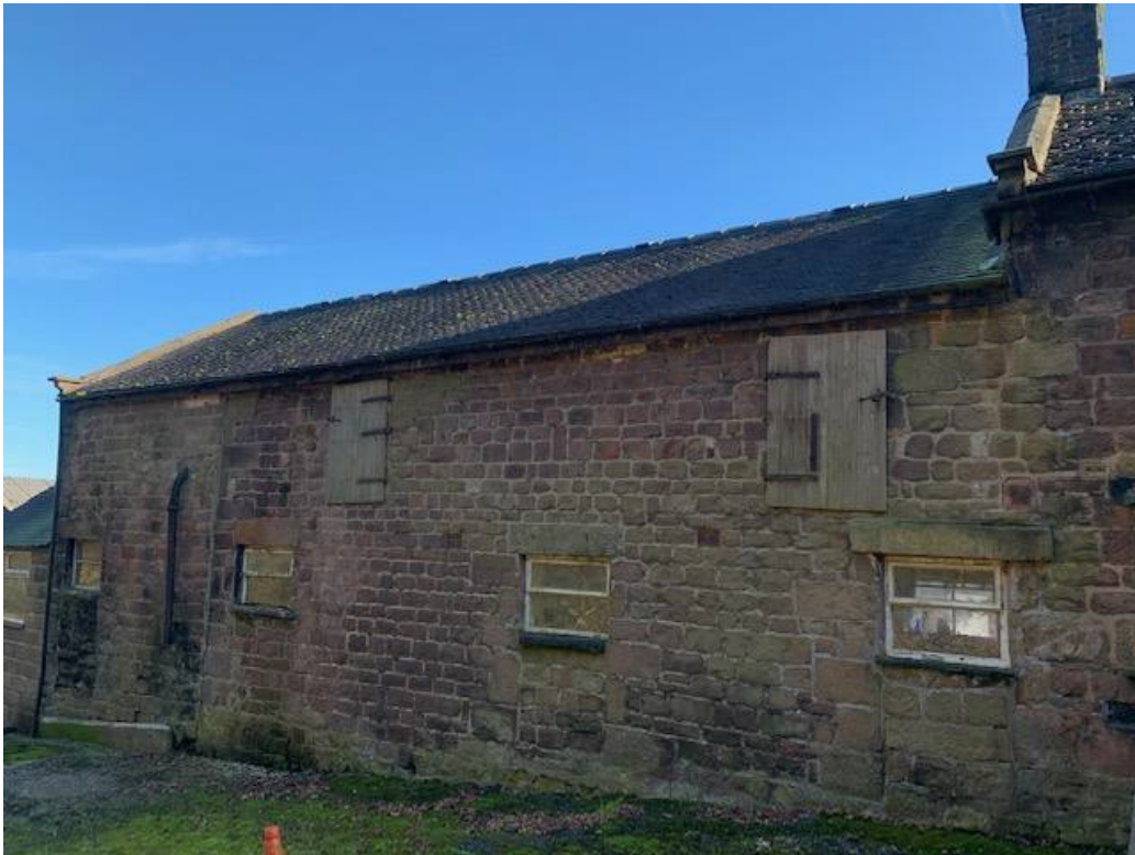
General view of west elevation of barn
