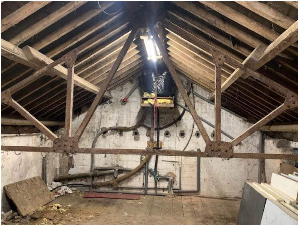
Typical internal view of stone barn showing timber purlins and steel truss.
