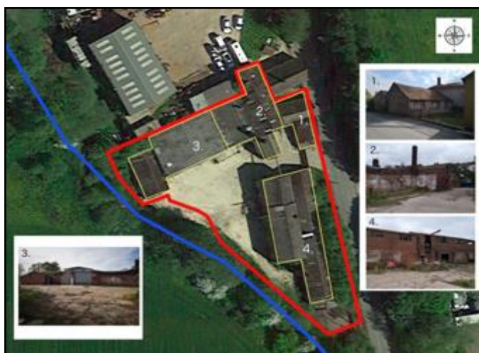
Figure 2. Aerial view of Adderley Mill buildings + associated hard-standing areas and boundaries in relation to watercourse.
