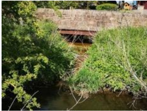
Figure 4. Bridge culvert side tributary.
