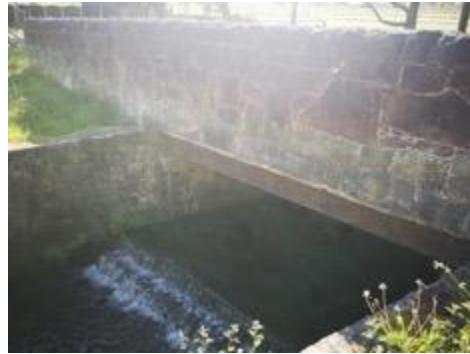
Figure 5. Main bridge underpass and weir.
