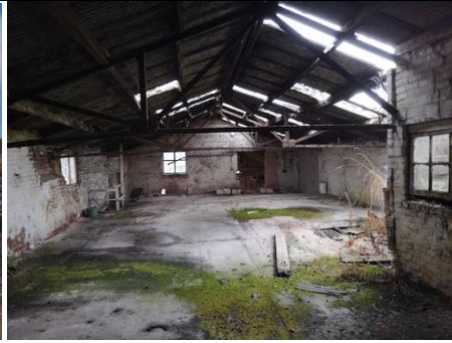
Fig. 9. First-floor region in main section of B2.
