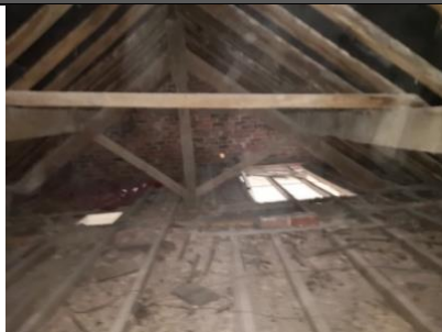
Fig. 5. Internal roof void area.
