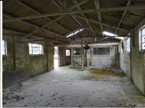
Fig. 13. Internal first-floor region of B4 .
