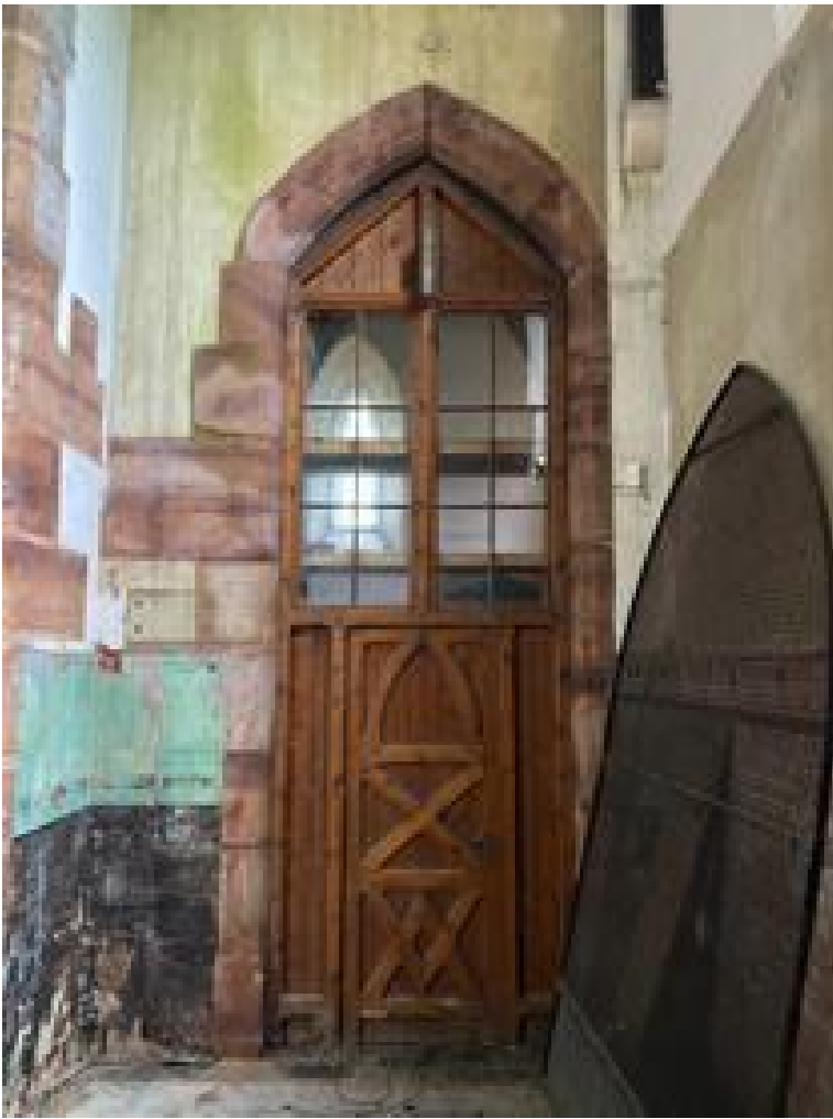
D7. Door and screen to Tower.
