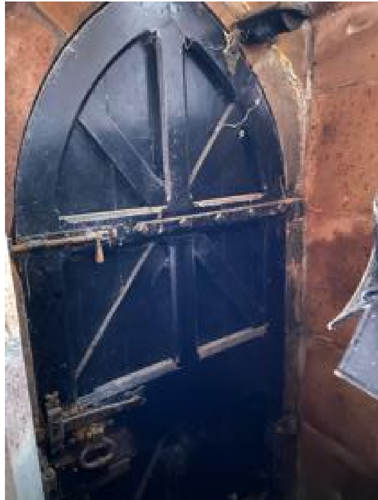
D1. South Entrance into Tower.
