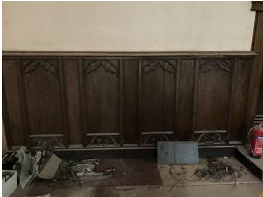
P. Gothic Panelling installed in 1928.
