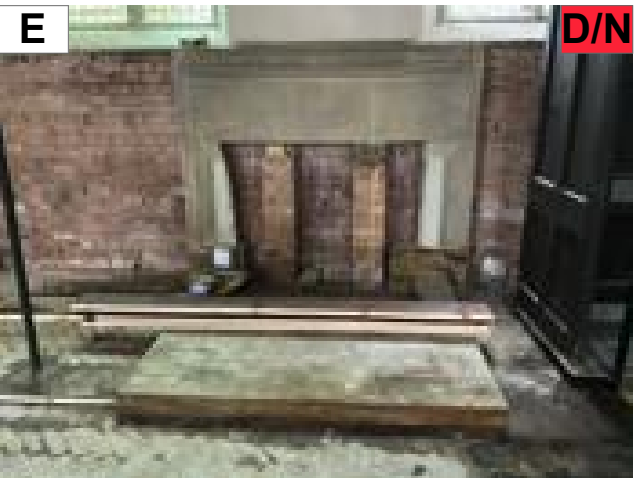
E. Reredos only of the Sacred Heart Altar 1932 (Drysedale) TO BE REMOVED AND RELOCATED.
