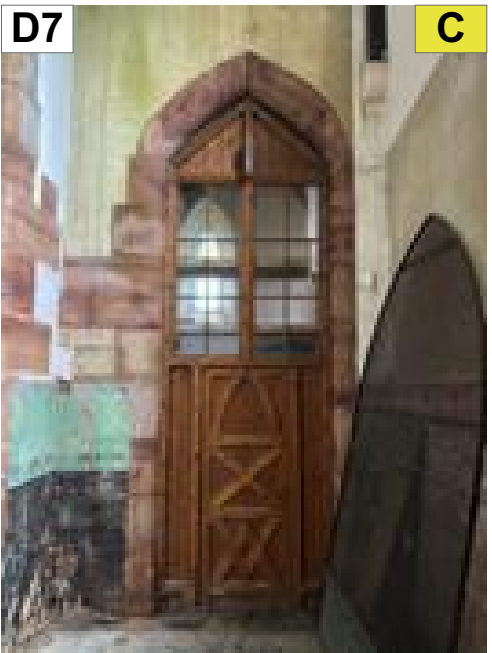
D7. Door and screen to Tower. TO REMAIN.
