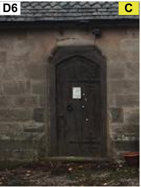
D6. Entrance into Cloister. TO REMAIN.
