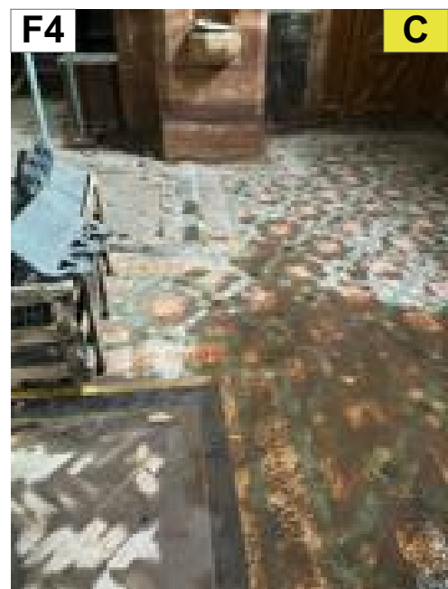
F4. Decorative tiled floor abutting woodblock floor around entrance door and tower buttress. TO REMAIN EXPOSED.
