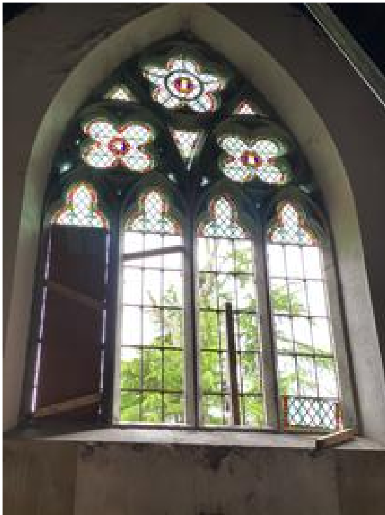
2. West Window - Stained glass removed by diocese.
