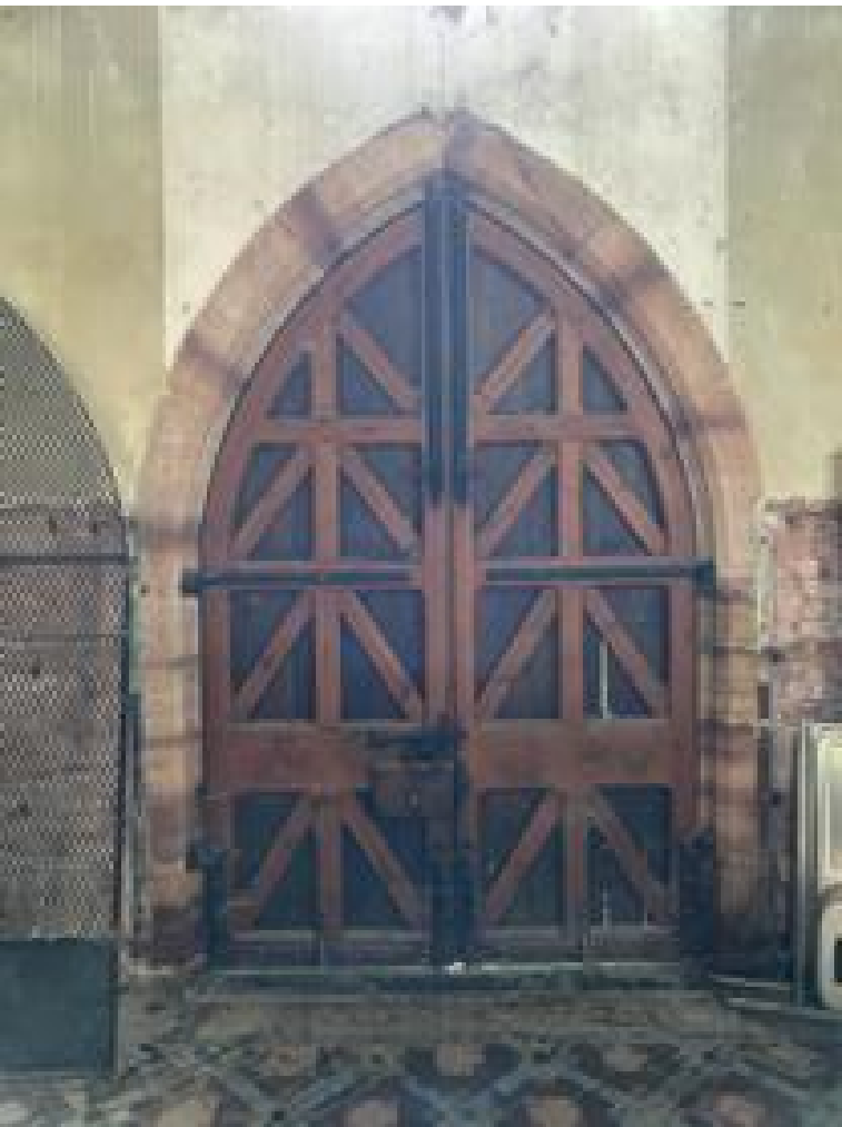
D4. West Entrance Door.
