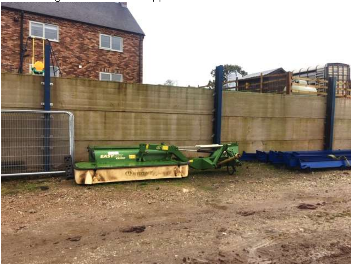
2. View showing existing garden retaining wall which would be used to support the proposed development
