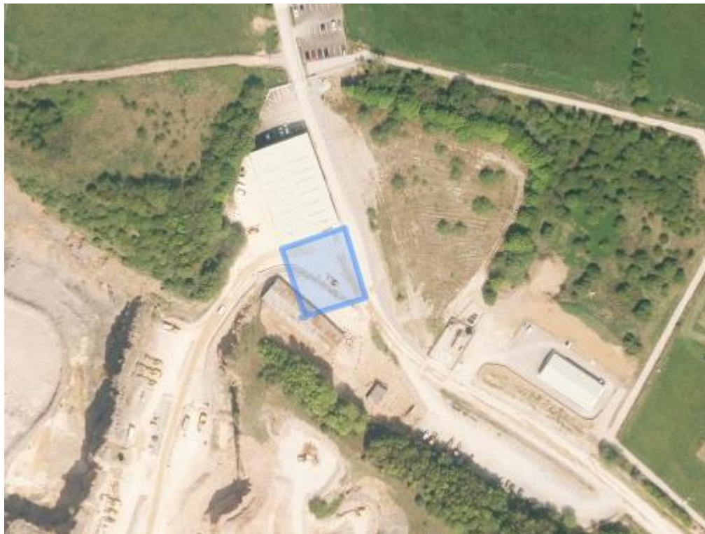
Figure 1: R&D Building extensions area 2
