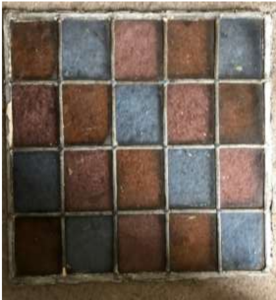
Fig H06: Handmade coloured leaded glass to be used in new door
