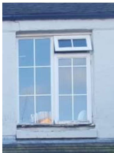
Fig H05: Existing windows ; single glazed storm casements with planted glazing bars
