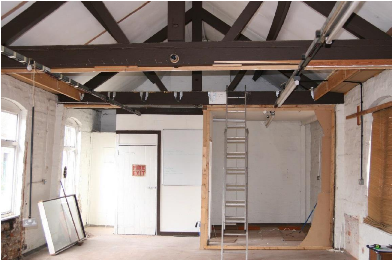
Figure 12 – timber major roof trusses (first floor, looking northward)
