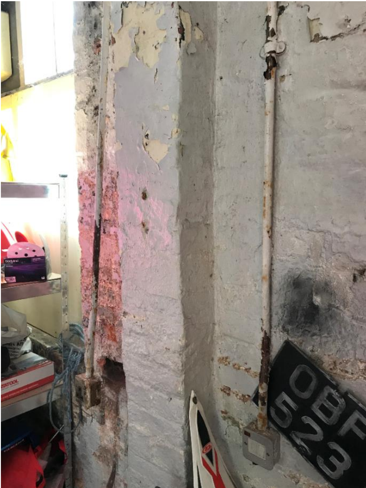
Figure 11 – typical masonry pier
