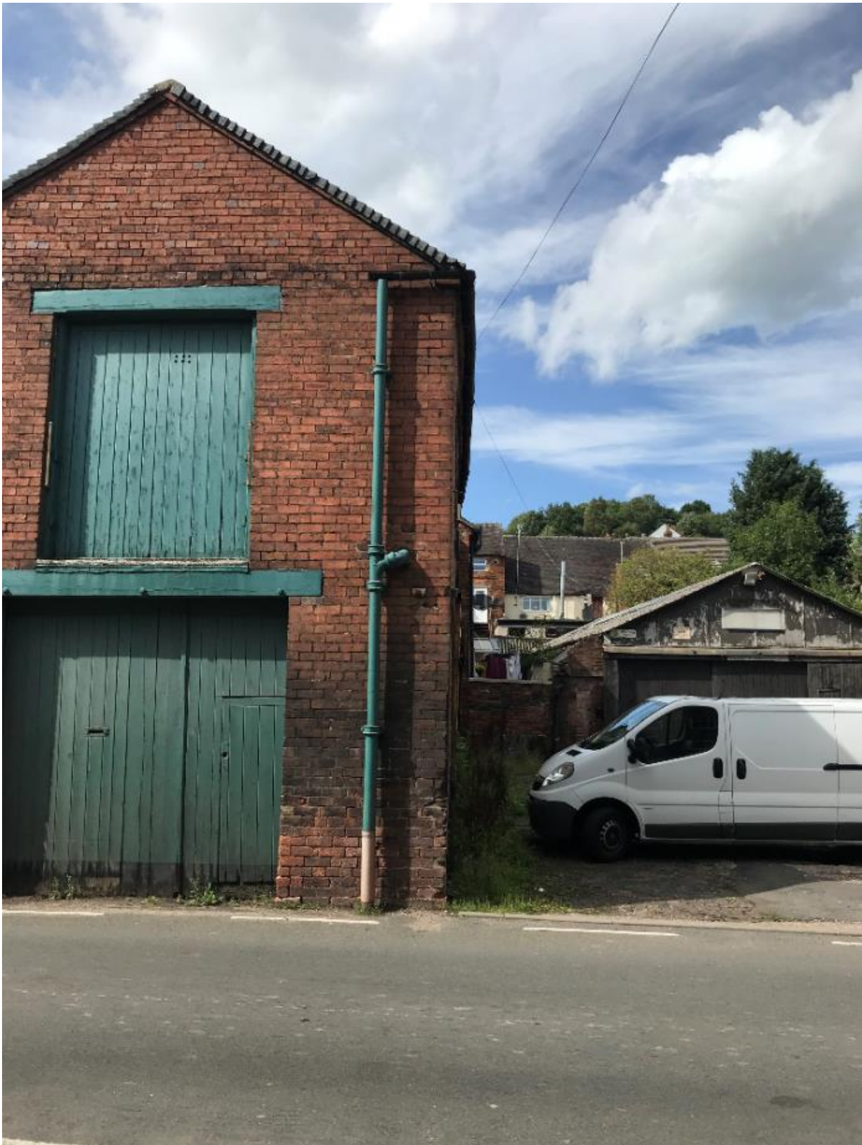
Figure 3 – gable elevation and rear yard
