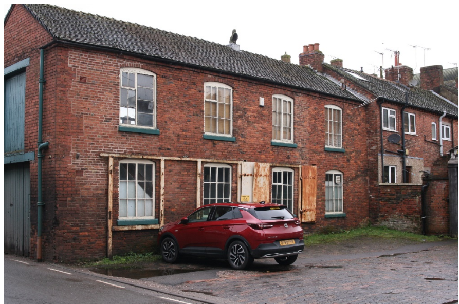
Elevation to garage parking area
