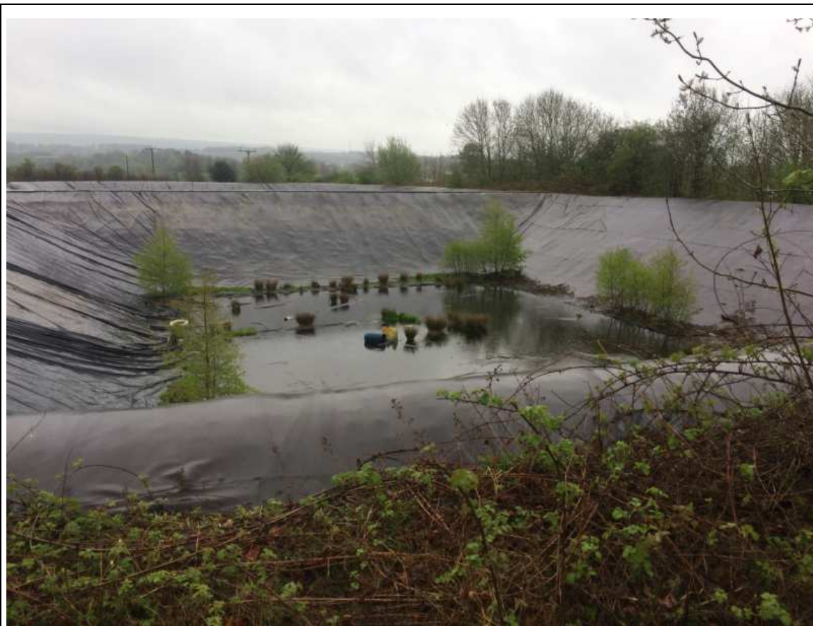
View of the storage pond showing liner.
