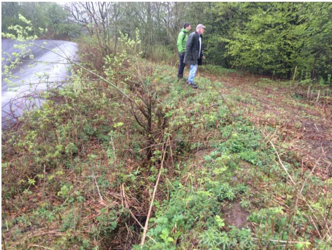
South east corner showing the falling ground to the lane below.
