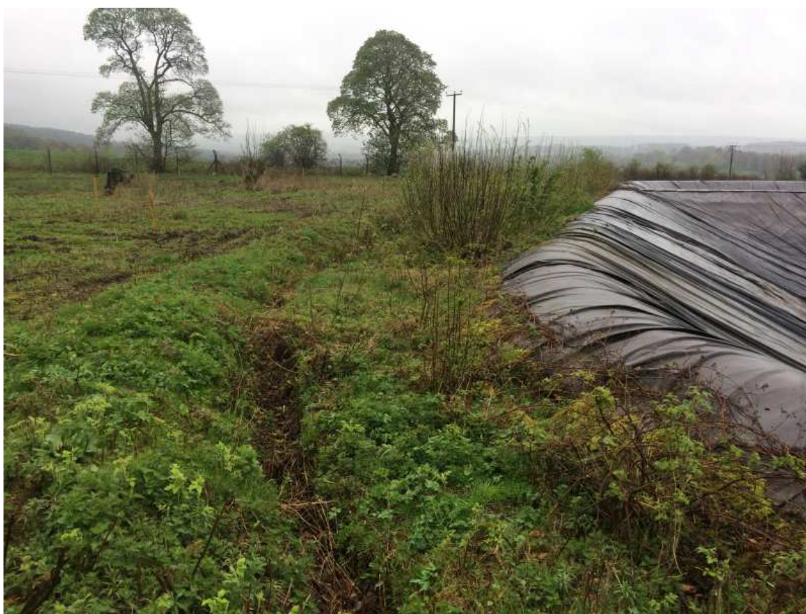
View of pond perimeter showing the wrapped liner buried at the endge.
