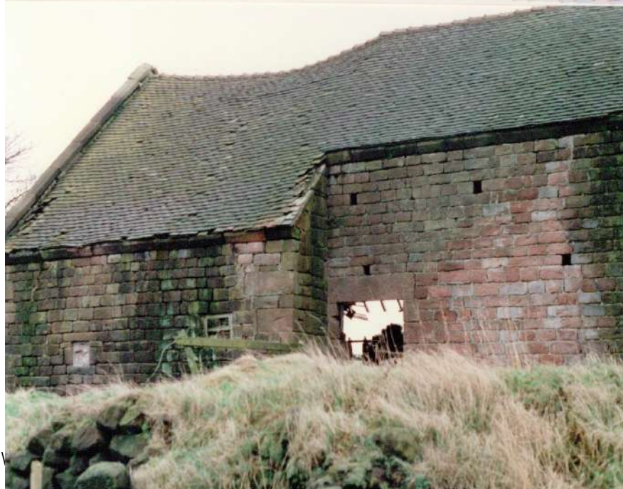
Fig.6 The northwest rear elevation of the barn just prior to the commencement of works in January 1992, showing the 'winnowing' door opening and sandstone lintel (source: client archive)
