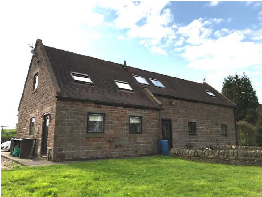
Fig.10 The Barn northwest rear elevation as it appears today (2018). Three of the openings on the elevation are largely 'as existing' and as approved. The far two windows and all of the large single-pane Velux rooflights are unauthorised ( photo: ctd architects )
