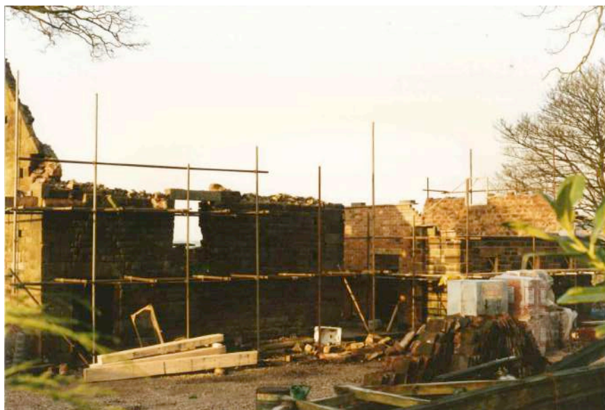
Fig.7 The southeast front elevation during the reconstruction of the roof and the two north end Bays (trusses are visible in the foreground) (source: client archive)
