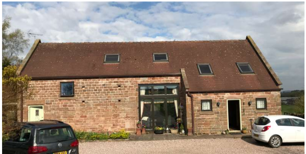
Fig.9 The Barn southeast front elevation as it appears today (2018). The openings on the elevation are largely 'as existing' and as approved, but the central pair of large single-pane Velux rooflights are unauthorised (photo: ctd architects)
