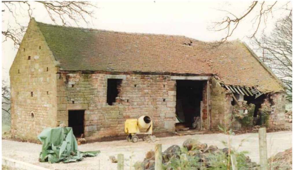
Fig.3 The southeast front elevation of the (north) barn just prior to the commencement of works in January 1992, showing the large cart opening, projecting later north out-shut and cow house at the south end, and vernacular character (source: client archive)
