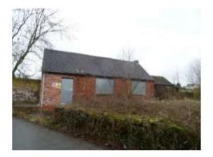
The cottage situated beyond a lane to the east of the site is brick constructed with a pitched roof supporting a combination of tiles and corrugated sheeting. The building is currently redundant and boarded across the windows but was considered to be in reasonable condition with the exception of a number of absent/slipped roof tiles. However, close up observations of the building exterior were not possible, nor was the interior of the building investigated due to restricted access.
