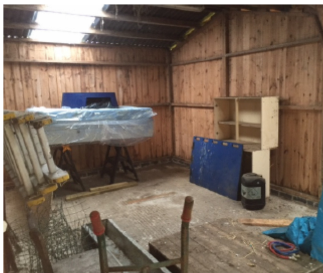
Timber frame and external cladding to be retained and lined internally
