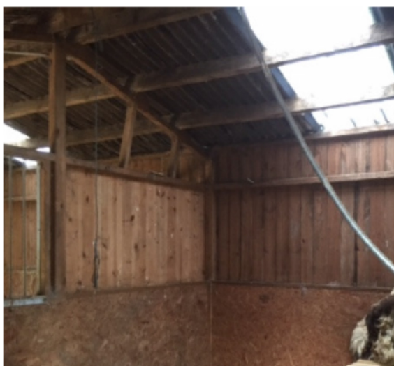
Timber trusses and purlins – to be retained
