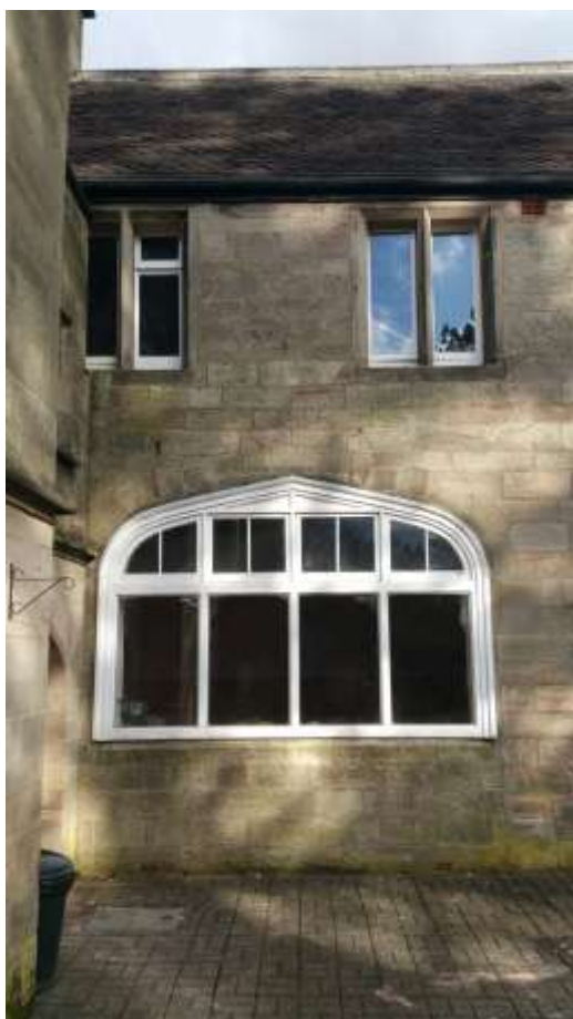
Figs. 40 and 41 The four centred arches to the partially blocked coach house doors
