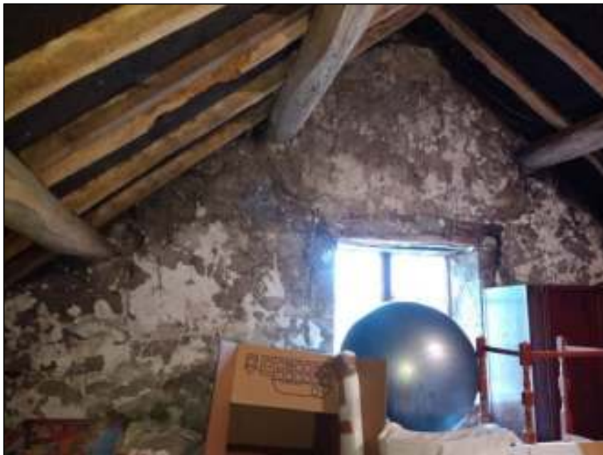
Photographic plate 6: First floor room showing the plater lined walls and window lintel
