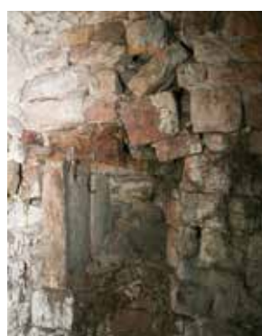
Window - to south wall recently blocked
