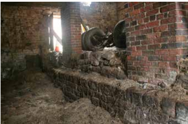
Left - coursed and mortared stone plinth (looking south), which would have supported a short timber-framed structure of posts and horizontal rails; sockets survive in the south wall. Right - the cowhouse looking north, with 19th century brick piers.
