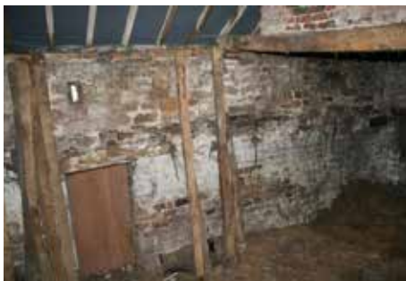
Oak posts (former joists) set aside. The sockets for the joists can still be seen in the masonry
