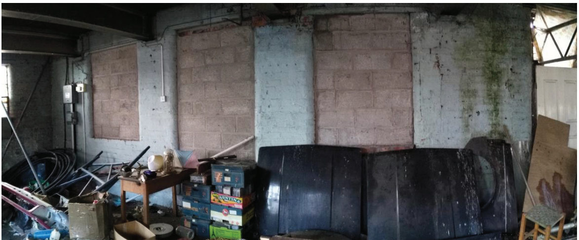
Figure 2: First Floor Wall between two “halves” of Britannia Mill
