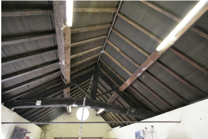
photo 4 - view of the king post truss
