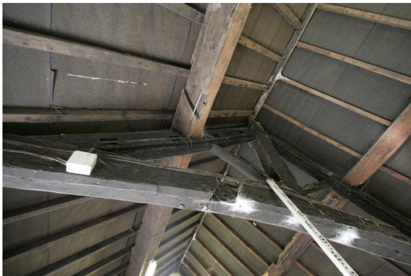
photo 5 - view of the king post truss
