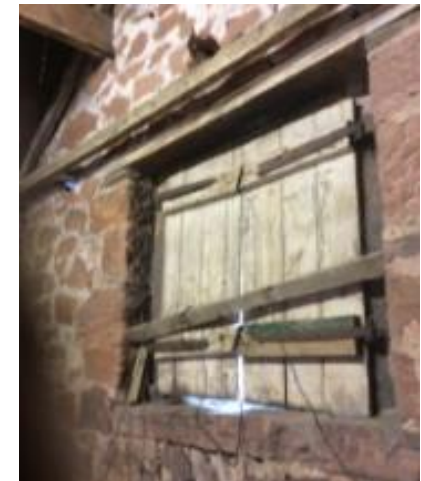
Photo 7: Boarded up window with gaps on the north elevation.
