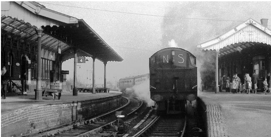
Illustration of the former Leek Station shortly before closure
