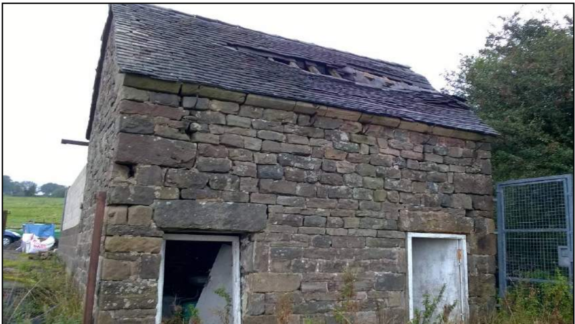
Plate 4 Building 2 from south, showing gaps in stonework
