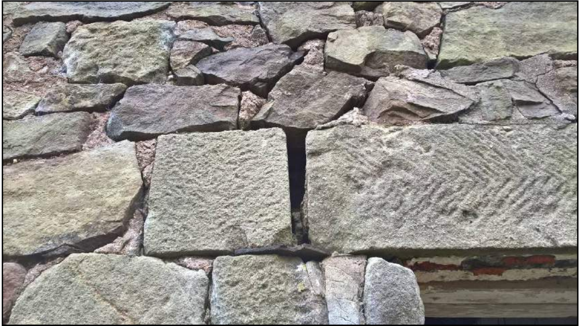
Plate 3 Building 1, showing multiple entry points to wall cavity
