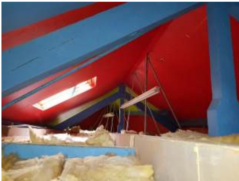
Plate 9: Showing internal roof void which shows boarded ceiling preventing full inspection.
