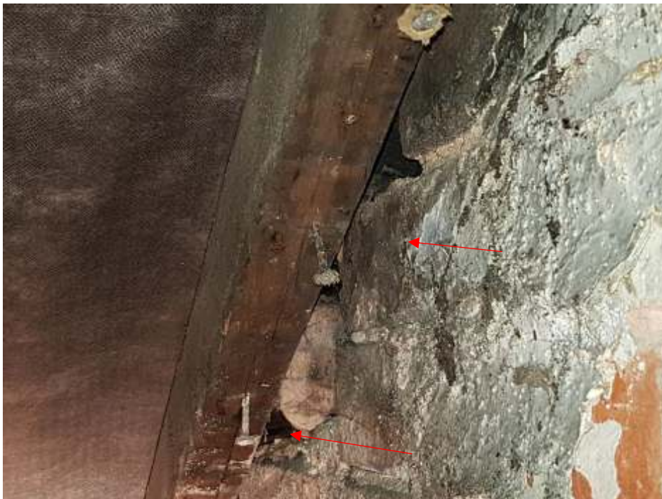
Plate 3: Showing potential roosting opportunity within the brick work
