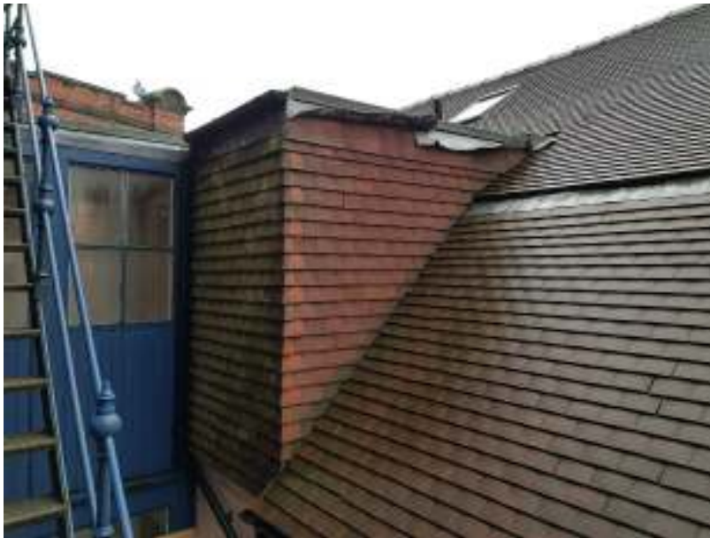
Plate 5: Showing drop down tiles which potential could provide crevices for bats to climb under.
