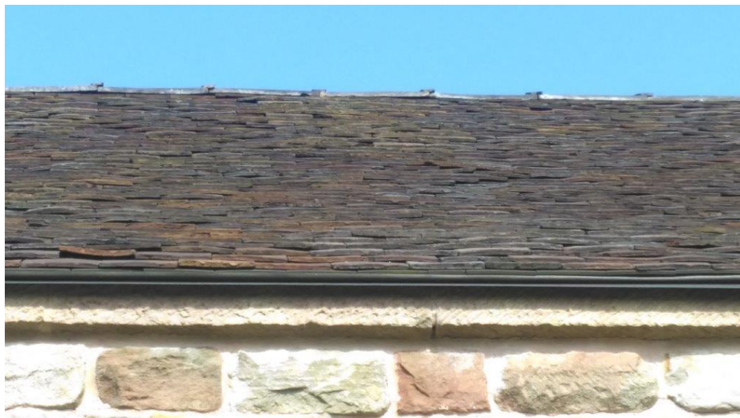
Plate 6: Gaps under ridge tiles and roof tiles of the barn (southern aspect) which could be used by roosting bats.
