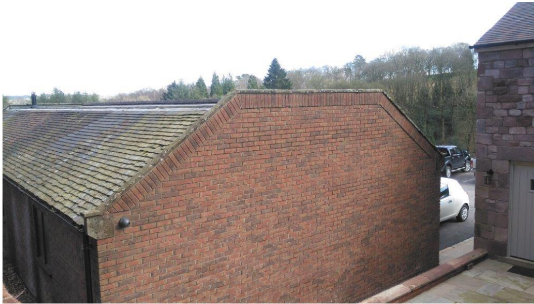
Plate 5: Northern side of the building showing the design of roof, with the central flat felt roof and the absence of soffits, eaves or bargeboards.
