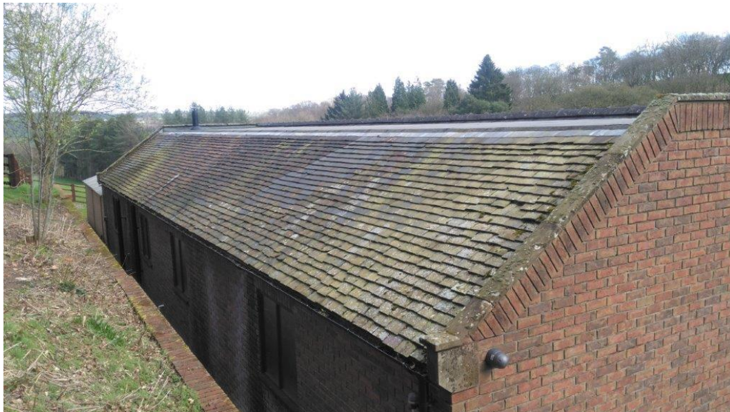
Plate 4: The western side of the roof with lead flashing and clay roofing tiles.
