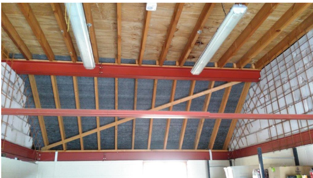
Plate 2: Internal structure of the roof with metal and wooden beams, lined with boards / breathable membrane.
