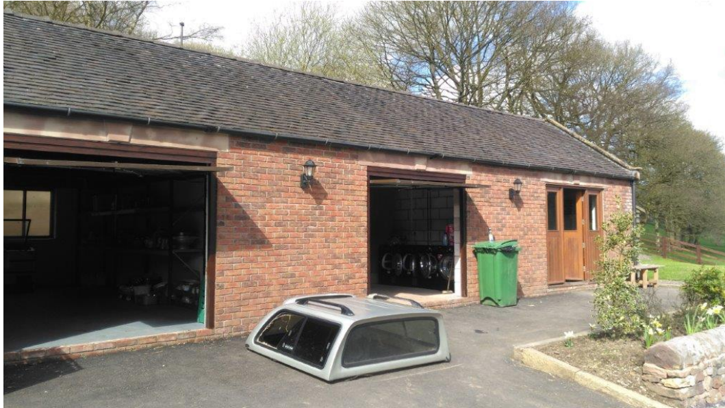
Plate 3: The roof of the outbuilding with 'ridge' tiles and clay roofing tiles (eastern aspect).
