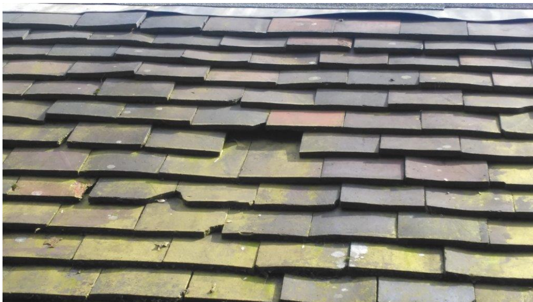
Plate 6: Example of missing tile and gaps under the lead flashing which could be used bats to access a roost between the tiles and membrane (western side).
