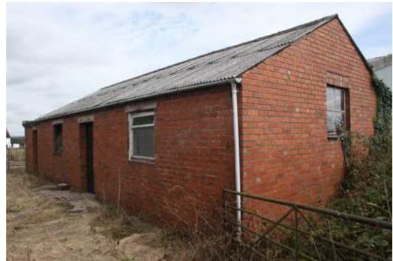
Image 6: Shows the north-west and south-west facing elevations of Building 2.
