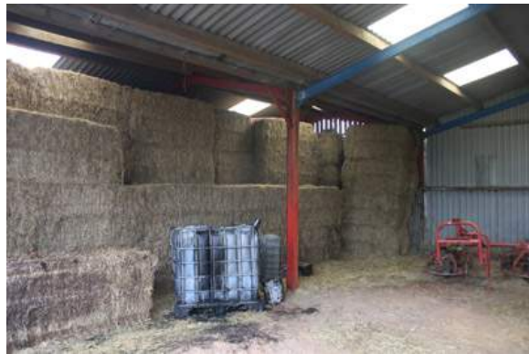
Image 4: Shows steel framework construction of Building 1 and stacked hay bales.
