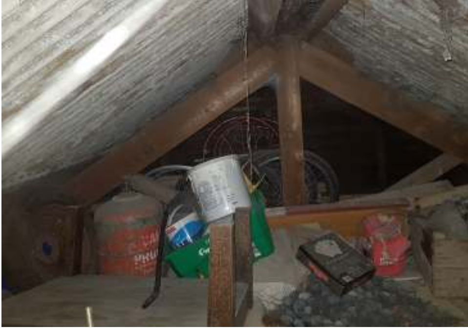
Plate 2: Showing the internal of the garage which provided limiting roosting potential
