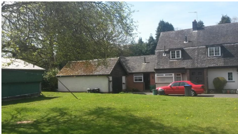
Image 3: Building partially within red line site boundary
