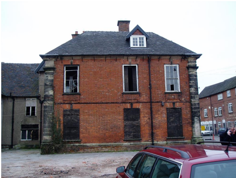
7: The rear of the Old Hall before restoration (Arrol & Snell Architects)
