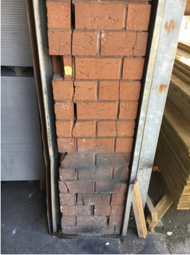
Photo 5 Cracked external wall
