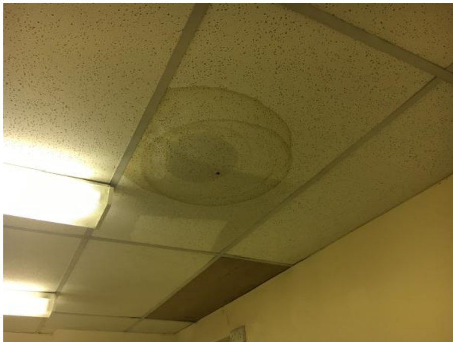
Photograph 8 Leaking roof
