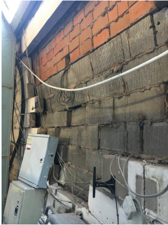
Photograph 7 Wall structurally unsafe
