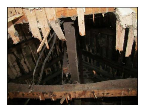
3.3.1.5. There is no felt beneath the roof tiles and therefore the slate laths and torching are exposed as shown below. There are areas where the torching has deteriorated and this has exposed various gaps. There are also gaps leading up beneath the ridge tiles and occasional gaps to the outside of the roof, particularly around the chimney at the eastern end of the roof.
