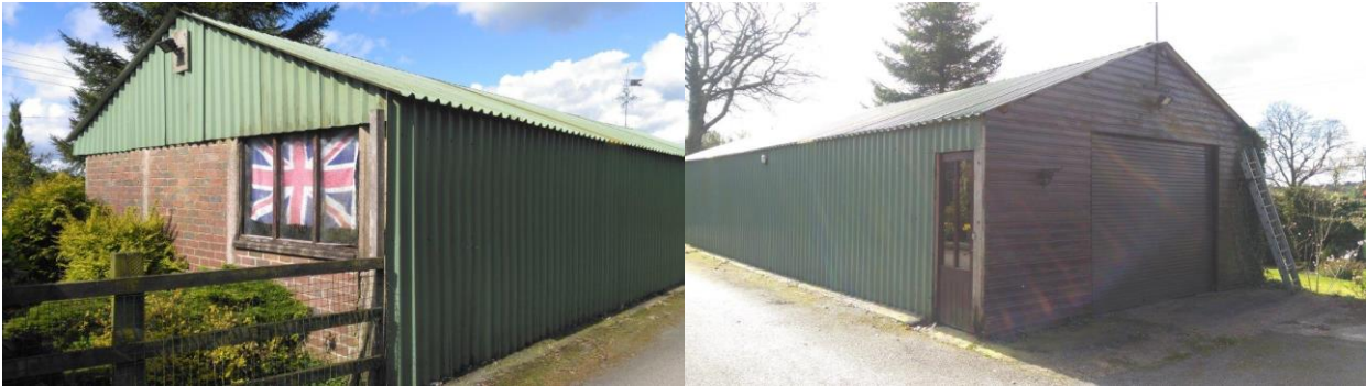
Plate 1: South end of building (Left); North end of Building (Right)
