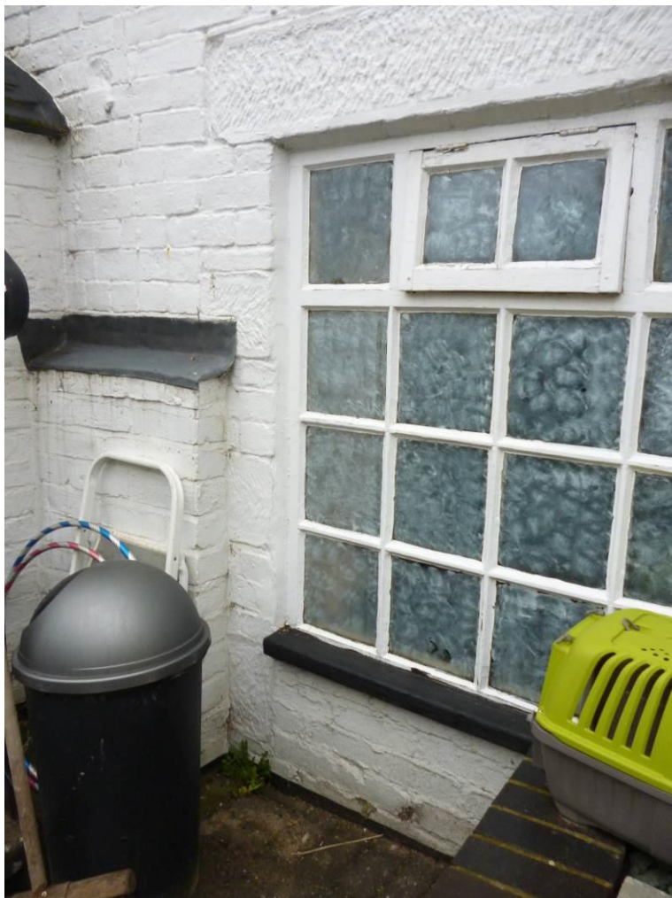
6: Detail showing original door opening below window
