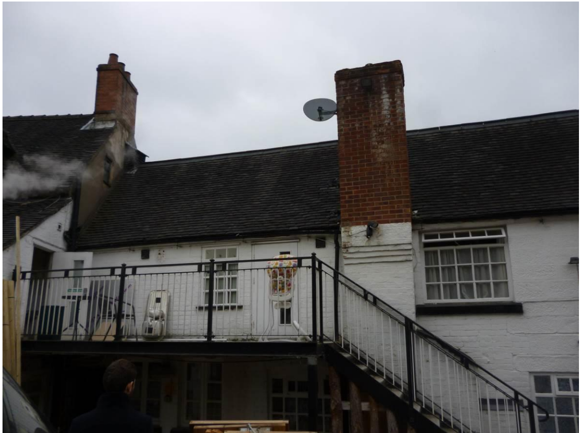
9: Chimney stack with modern brickwork
