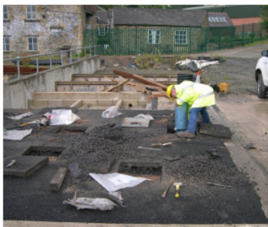
Figure 3 - In situ density tests post-trafficking.
