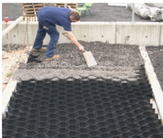
Figure 2 - Cellweb TRP® in construction.
