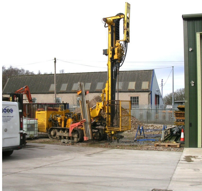
Drilling borehole R3
