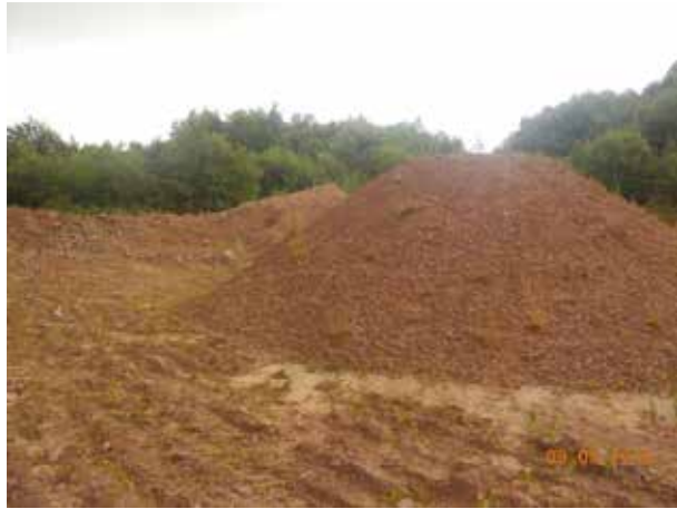
Plate 8: View of spoil mound (TN7)
