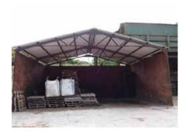
1.10 This was a steel framed single storey open fronted shed which had partially clad walls.
