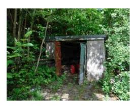
1.12 This building was a small single storey block built pump house adjacent to a reservoir. It had a flat felt covered roof that was in a poor condition.
