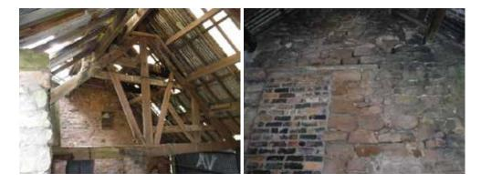
1.15 There was a part corrugated sheet metal/corrugated sheet asbestos/tile roof and a loft floor in one area.
