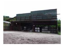
1.7 This was a two-storey steel framed and corrugated sheet metal clad building. The ground floor was used as an open storage area. The first floor was enclosed with walls with the roof clad in corrugated metal sheets.
