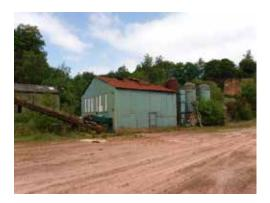
1.11 This steel framed single storey shed was clad in corrugated sheet metal..
