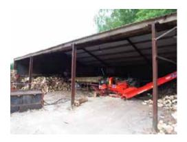
1.8 This building was a long steel framed single storey shed clad with corrugated metal sheets but open along its entire frontal elevation.
