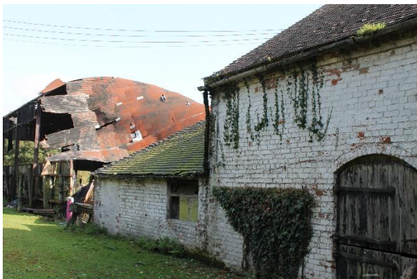
Barns 1 & 2 South Elevation (Western end)
