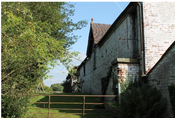
Barns 1 & 2 South Elevation (eastern end)
