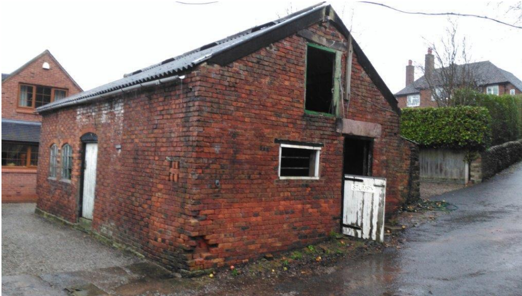
Plate 1: South aspect and east facing gable wall of outbuilding
