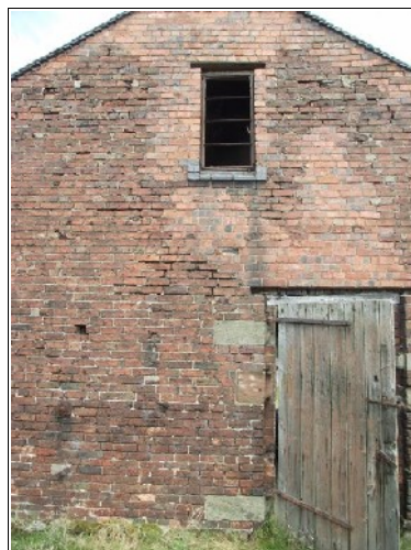
Fig.5. East gable-end of two-storey section
