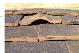
Fig.12. Examples of bat access tiles and soffit slits
