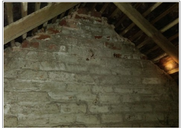
Fig.9. NE gable-end roof void
