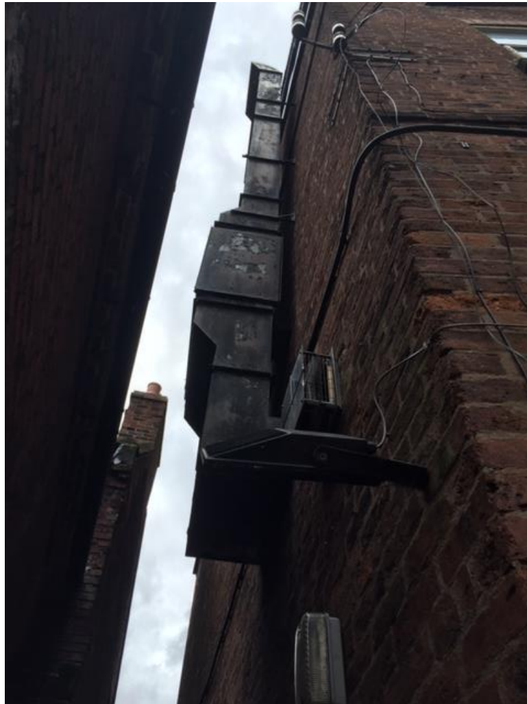
Image 1: Existing extraction duct
