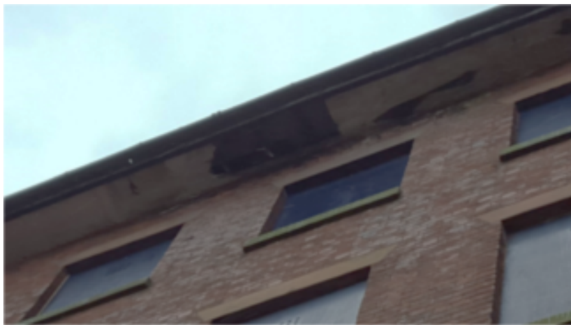
Plate 2: Showing missing section of soffit area potential access for bats & Birds.
