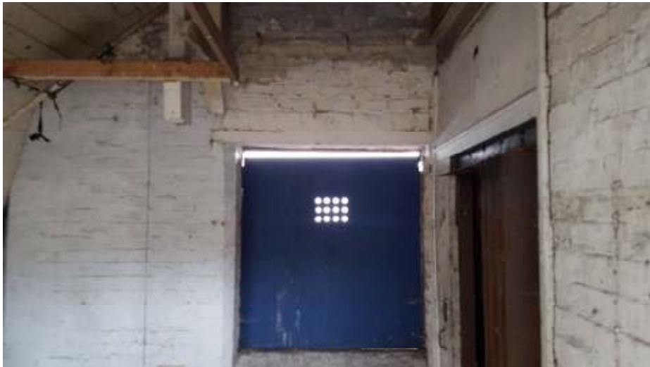
Plate 7 Showing potential access point through 2-5 inch crevices between the brick and window boarding, picture taken from level 3.
